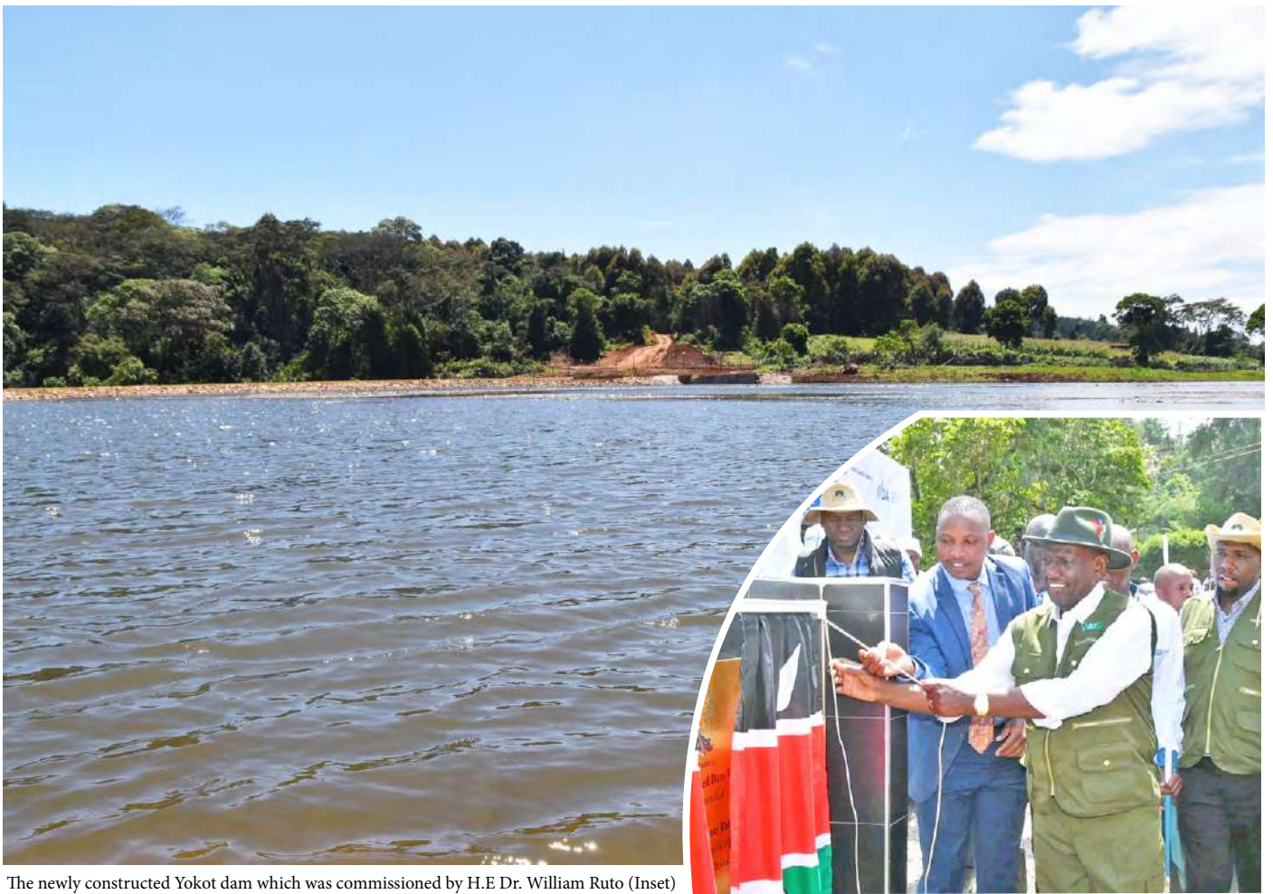
The newly constructed Yokot dam which was commissioned by H.E Dr. William Ruto (Inset)
